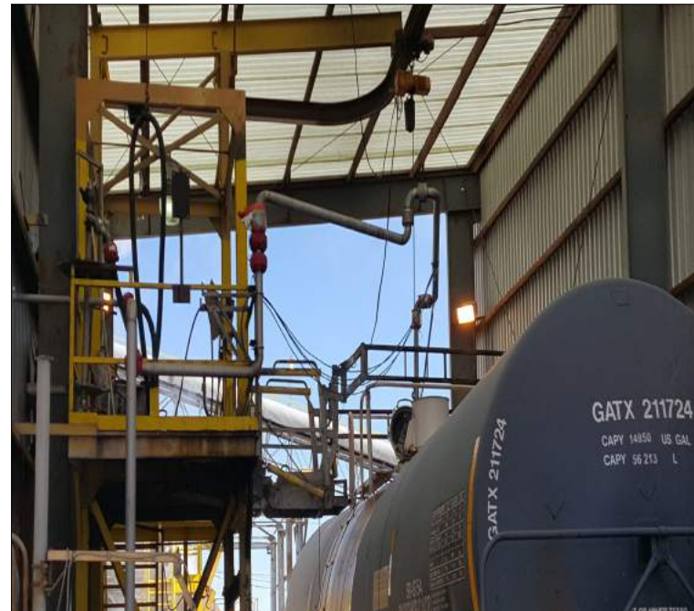
After: Engineered stainless steel pipe arm
