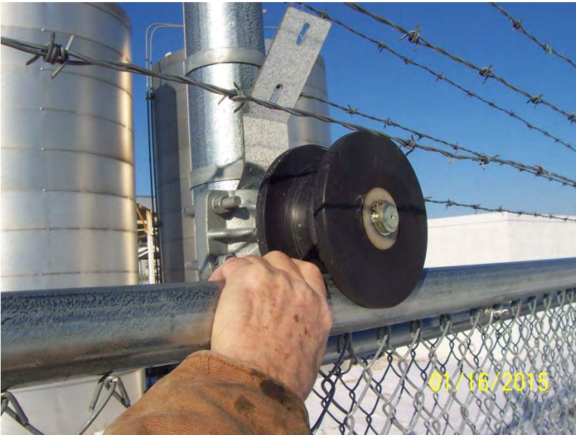
Gate roller assembly pinch point
