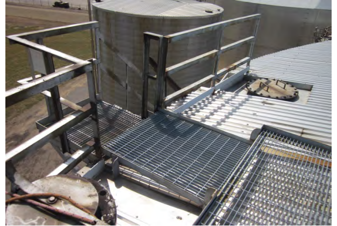
Old Tank Roof Platform
