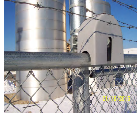
Gate roller assembly with Guard
