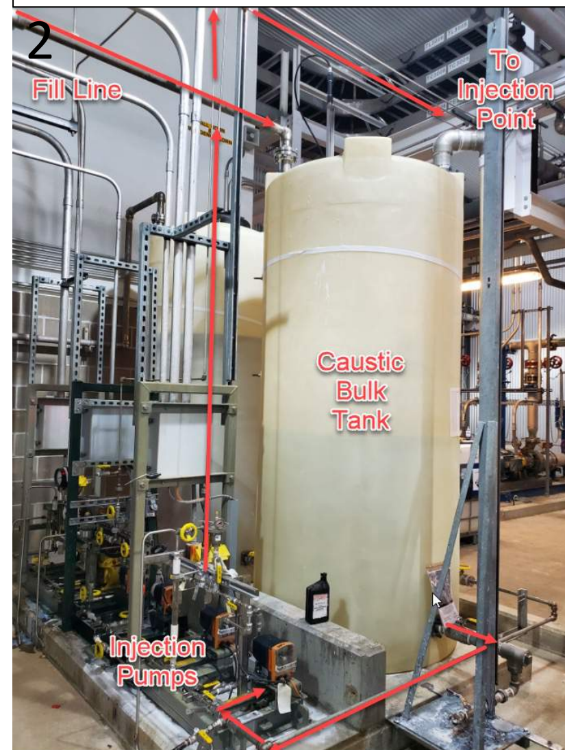
2. Caustic fill line, bulk tank, injection pumps, and pump discharge to the injection point.
