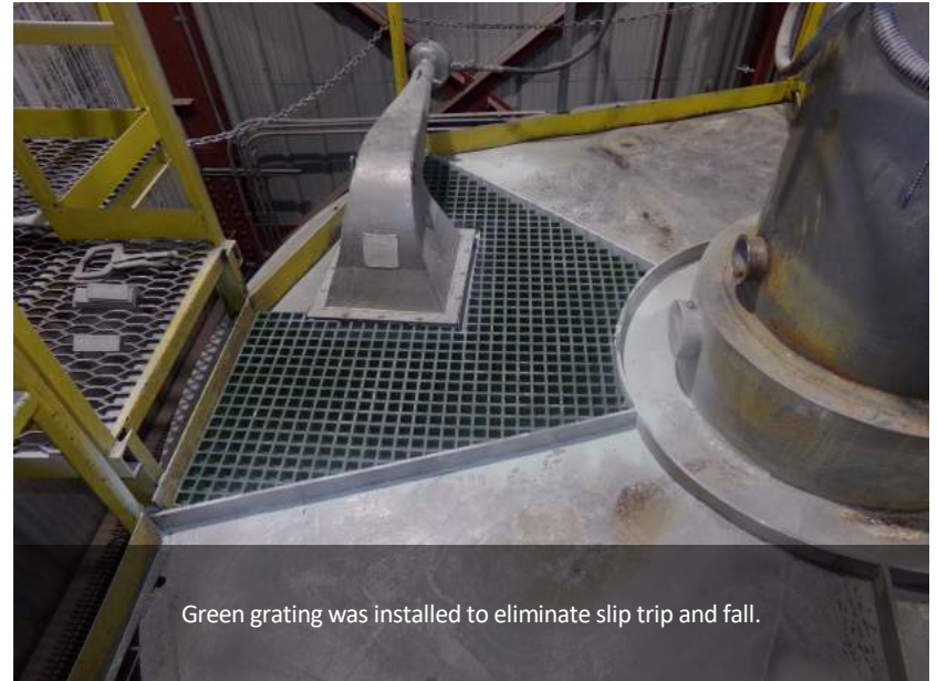
Employee walked on smooth metal surface. Would become slick if was wet.
