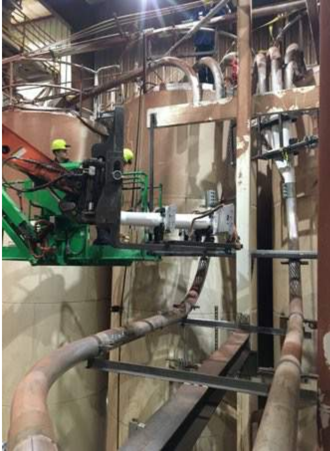
Pneumatic Valve installation
