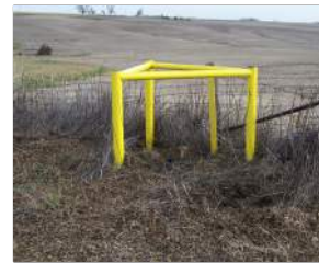
Barriers prevent the vulnerably exposed portions of the pipeline. (actual photo).
