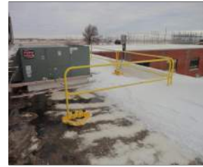
A fall protection system was installed (actual photo).
